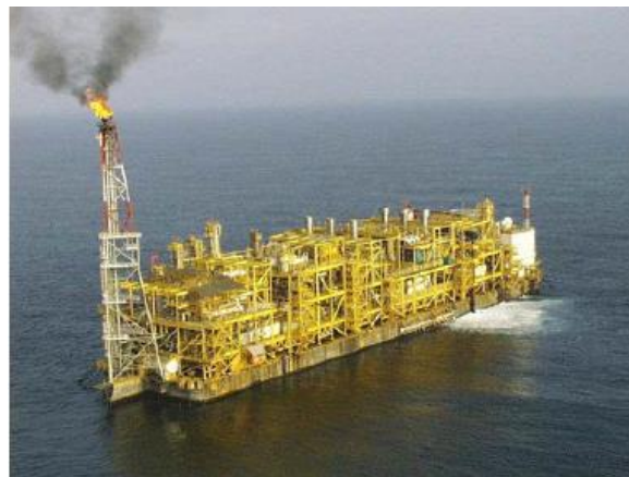
Figure 7 - N’Kossa field facility from Shokraneh et al. (2016)
