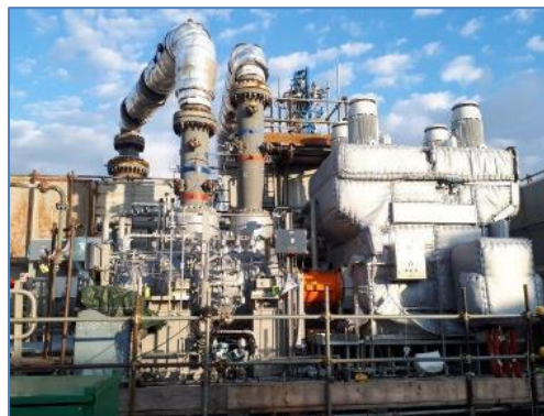
Fig. 1: Oil-free high-speed motor-compressor
