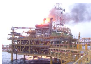
Figure 6 - Fire ignition due to DGS failure
