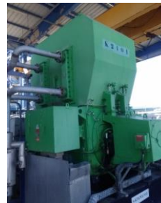
Figure 8 – Donges High Speed Motor fitted with AMBs
