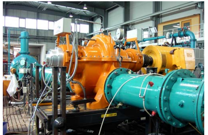
Fig. 4 Pump SM 400/400 in the Flow Loop Test Setup at KSB
